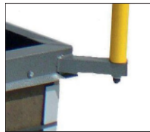
Rail Supports are Welded to Curb
